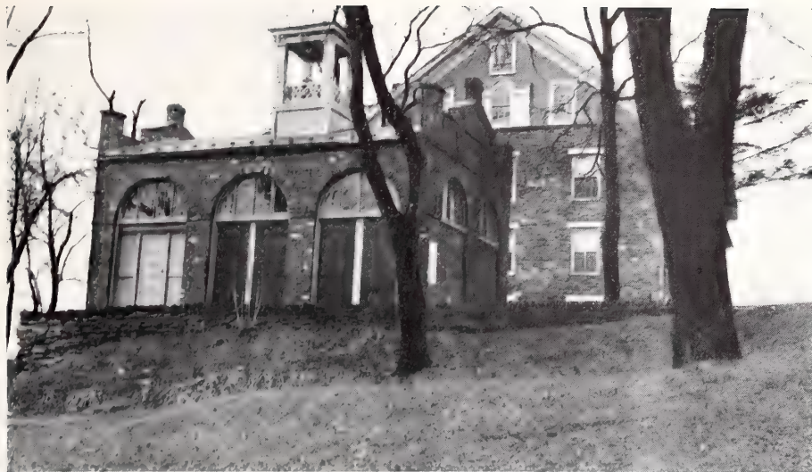
THE OLD BRICK ENGINE HOUSE, "JOHN BROWN'S FORT," ON ITS PRESENT LOCATION AT THE SOUTHWESTERN SIDE OF THE CAMPUS OF STORER COLLEGE, HARPER'S FERRY; PHOTOGRAPH MADE JANUARY 4, 1939.
